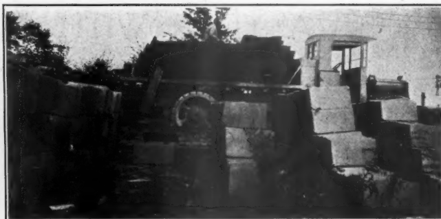
Truck Loading Roofing Slate at Storage Yard
